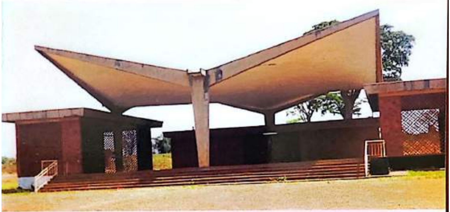
The Gymnasium at Busitema Campus
